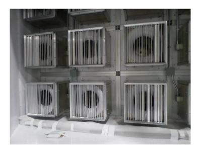
Coplanar silencer(s) and/or sound attenuator(s) shall be provided to meet specified acoustical requirements. Sound attenuator cross sectional area shall be selected to not exceed 500 fpm. Losses from sound attenuating devices must be included in the fan performance selection.
