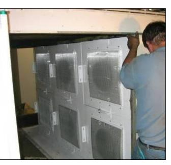
Stack FANWALL cells in any shape
